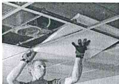
Figure 4: Installation of suspended ceiling
