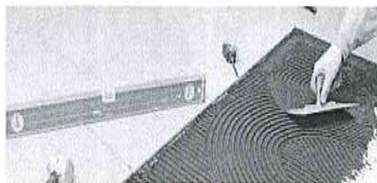
Figure 9. Ceramic tile application
